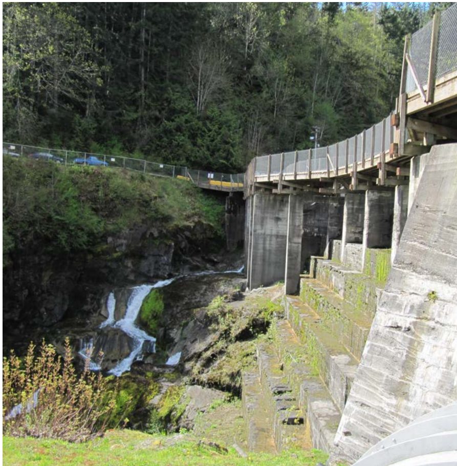
Before and after the dams were removed
